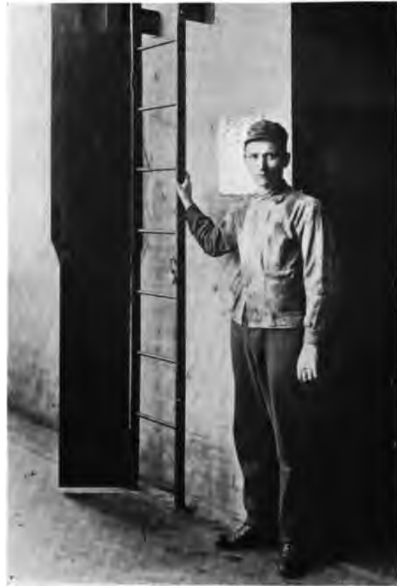
Fig. 2. Fixed Ladder with Locking Door.*
